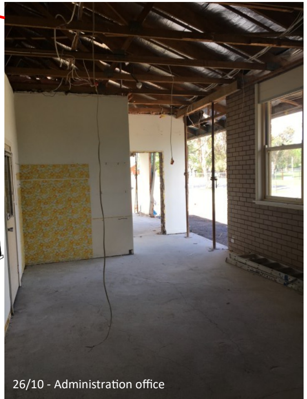
12/10 - Demolition of store rooms
